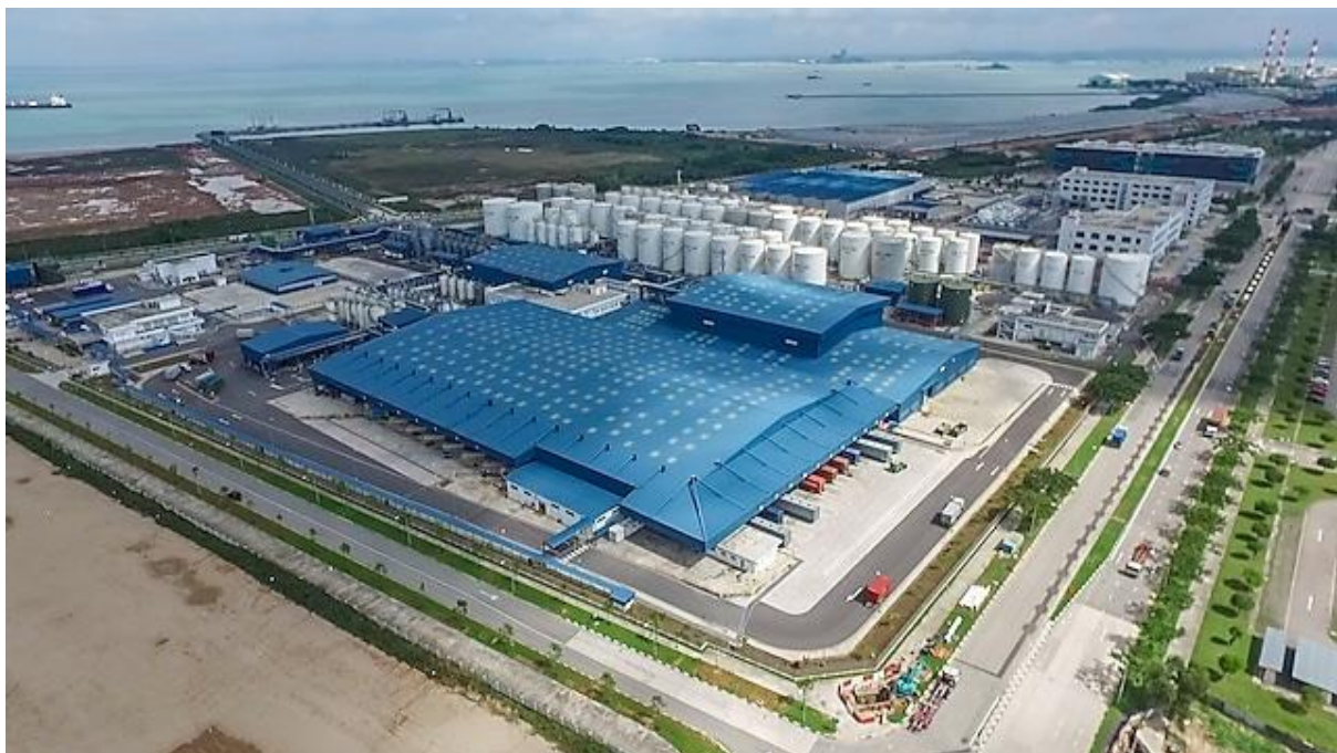
Shell Tuas Lubricants Plant
